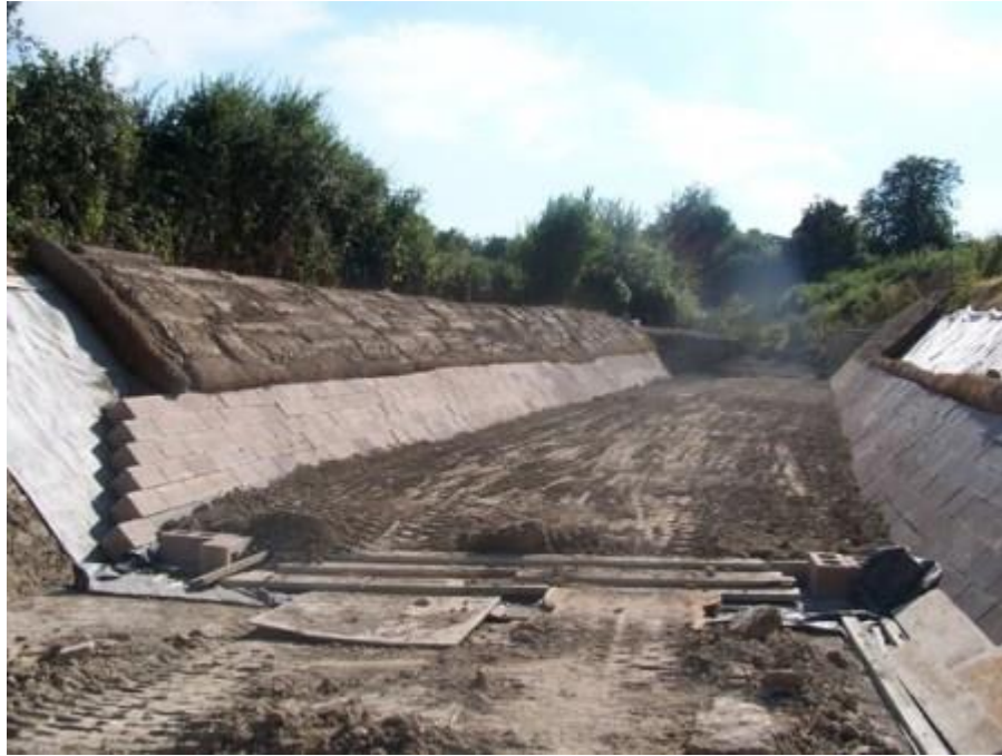
Fig 5: Construction of Brick Canal Lining
