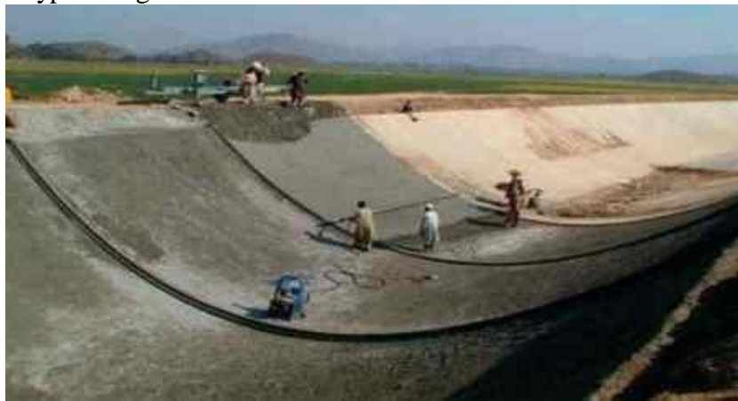
Fig 4: Cement Concrete Lining
